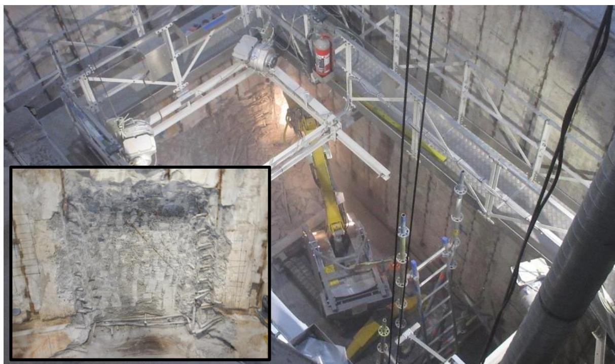
**Figure 7: top view of the BR3 biological shield showing the BROKK pneumatic hammer used to remove materials from the test section. In-frame picture: close up of the curved wall after partial material removal**
